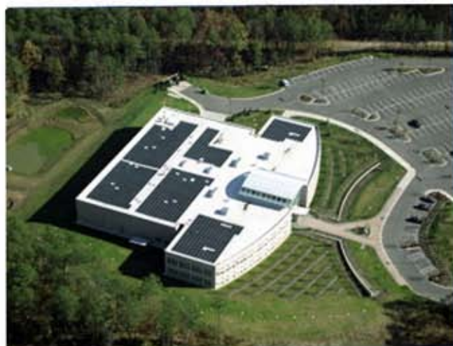
Photo 4 – One of the more prominent buildings that combines a cool roof with solar panels is the EPA’s 101,000-sq-ft National Computer Center in RTP, near Raleigh, NC. Photo courtesy of the EPA.
