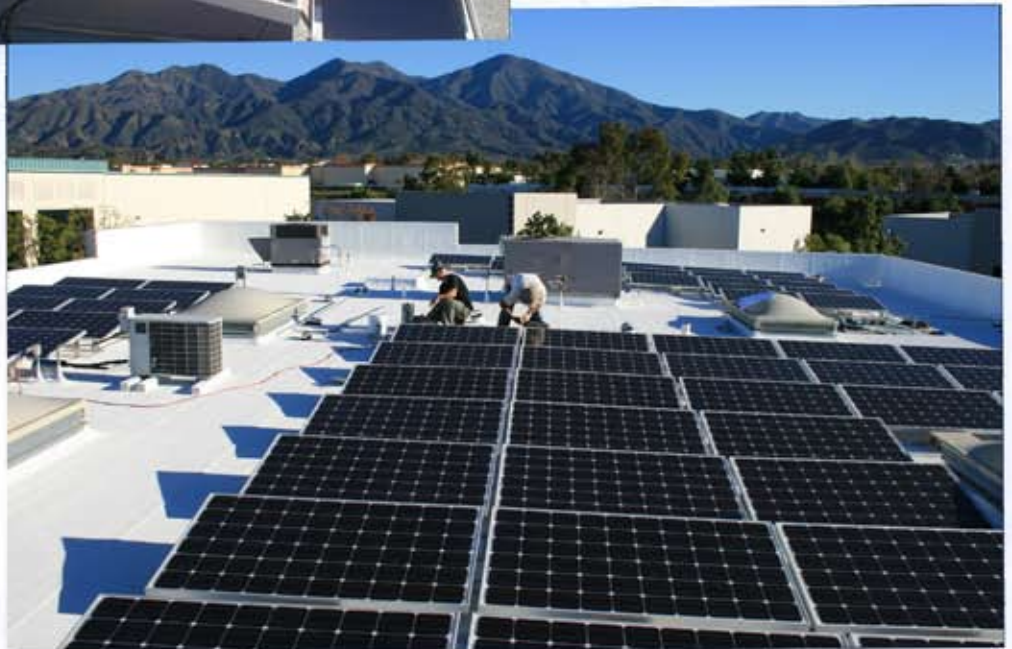
Photo 3 – Energy-efficient cool roofing systems can significantly reduce roof temperatures during the summer, improving the performance of the photovoltaic system. Photo courtesy of Coat’N’Cool.
