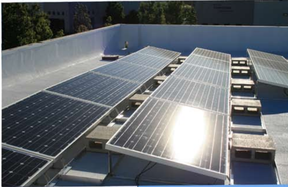
Photo 2 – A cool roof as an integral component of a solar installation enhances reflectivity and other benefits, such as cooling a building’s interior and helping to improve the operation and efficiency of the photovoltaic system. Solar systems work best at temperatures below 90°F. If temperatures exceed 110°F, the solar power output can be reduced by as much as 50%. Photo courtesy of Coat’N’Cool.
